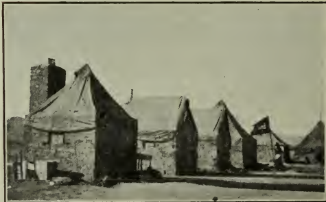
FIG. 8.—Pyramidal and hospital tents erected on adobe walls.
